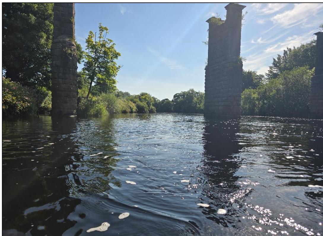
Figure 3-2 - Depositing/lowland rivers (FW2) habitat at proposed River Finn crossing in Ballybofey/Stranorlar (Ch. 29500).
