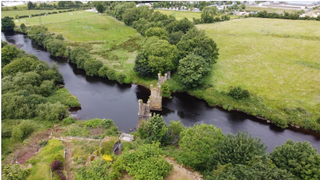
Figure 4-8 - Existing Railway Piers in River Finn (S20)
