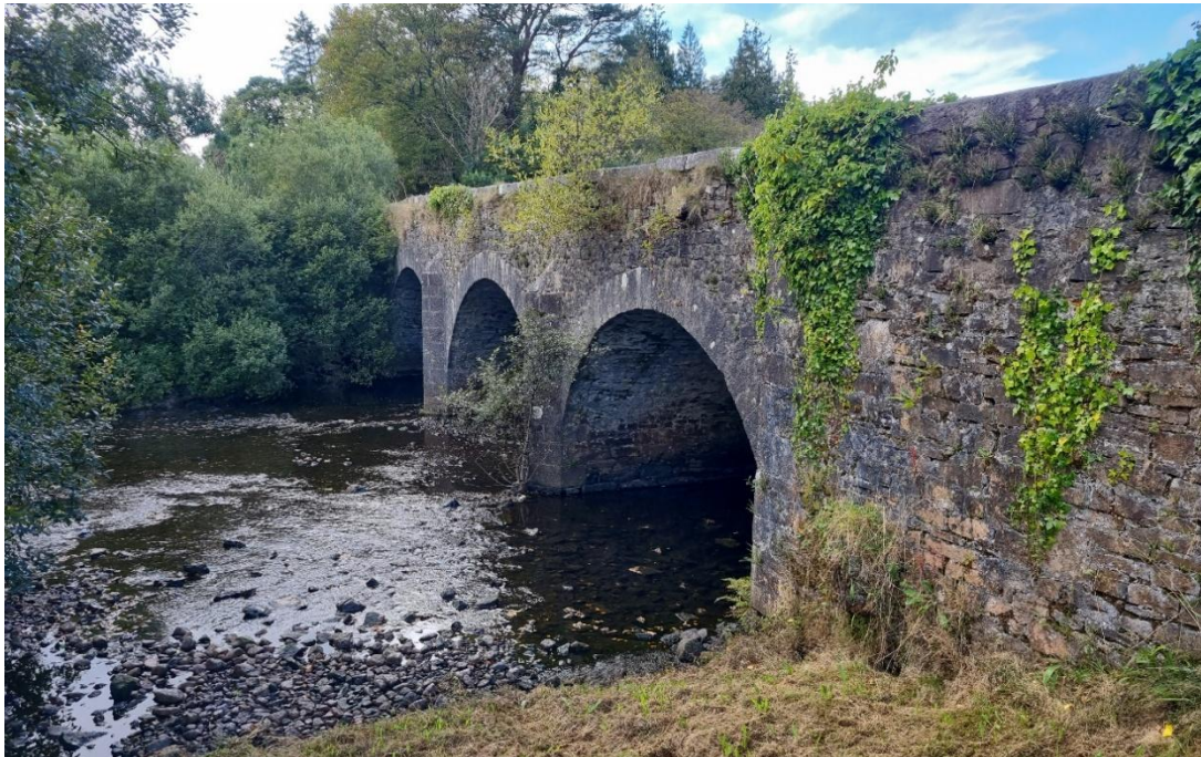
Figure 4-4 - Existing Road Bridge over River Eske (S05)
